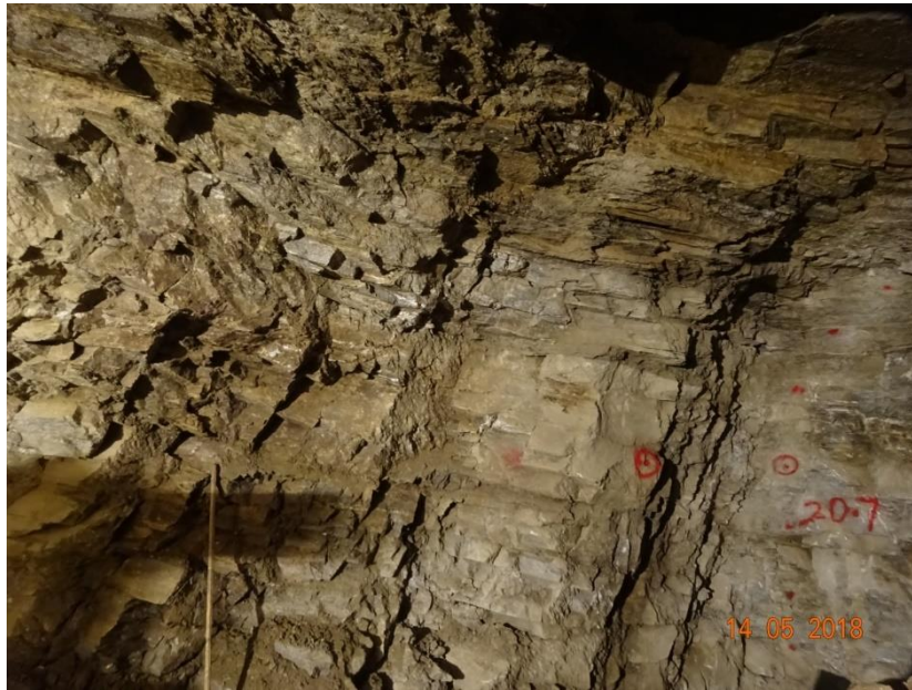
Figure 4-29: Rock Mass observed in the Test Adit
