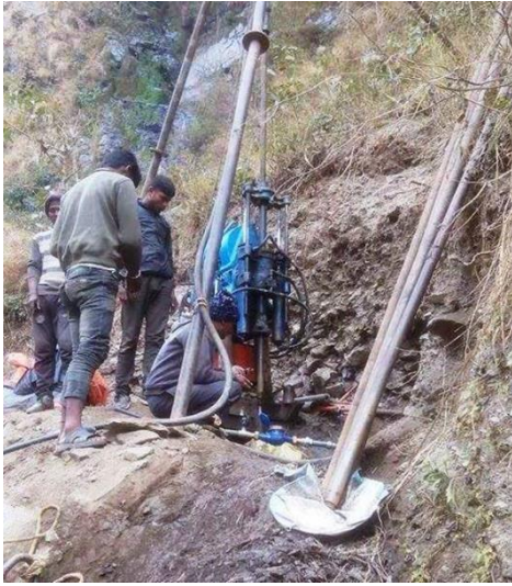
Figure 4-23: Core Drilling being Operated in Borehole SW – 1
