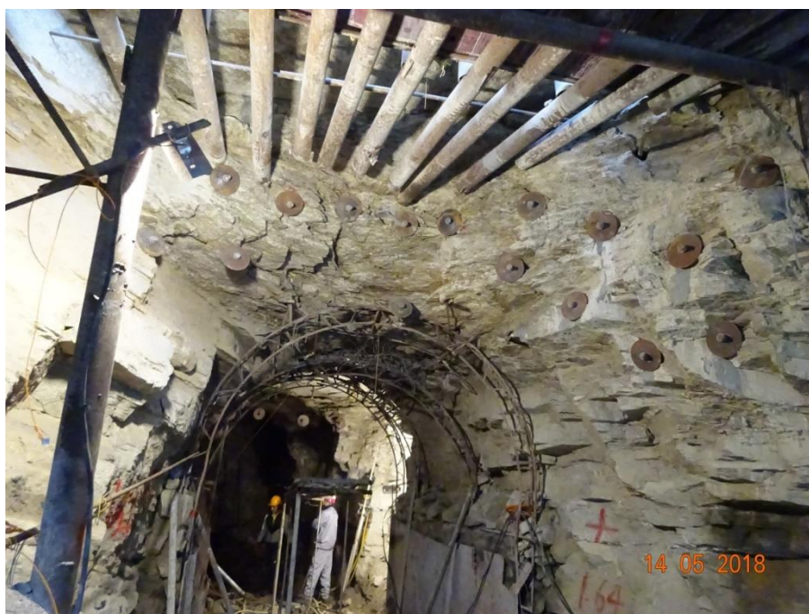
Figure 4-30: Installed Support in Test Adit
