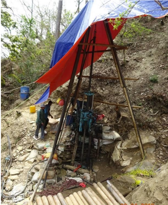
Figure 4-25: Core Drilling Being Operated in Original Borehole HB – 1'
